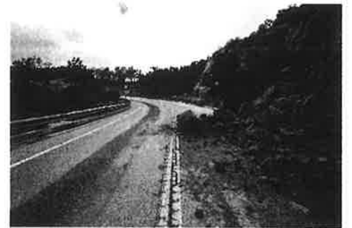
Landslide over a highway in Southern California
